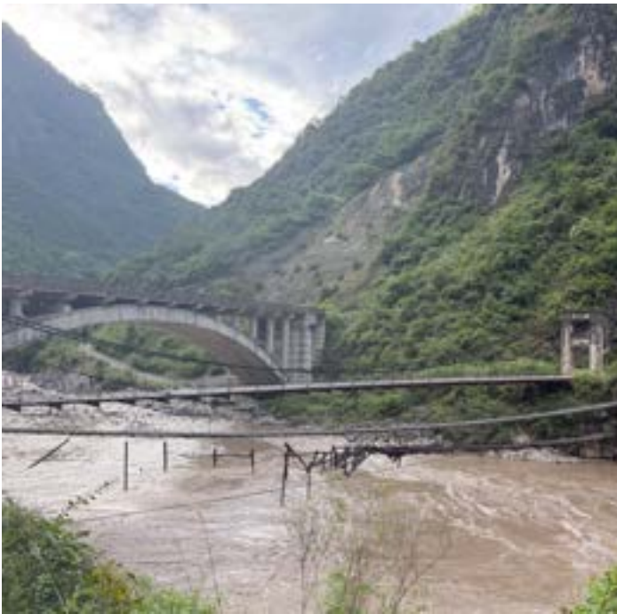
Multiple bridges crossing the Angry Nu River
